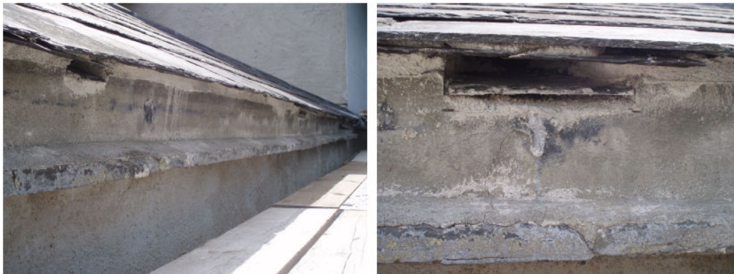
Figure 9: Artificial roost access slits under eaves suitable for Pipistrelle species (Bishop's Palace, Kilkenny)
