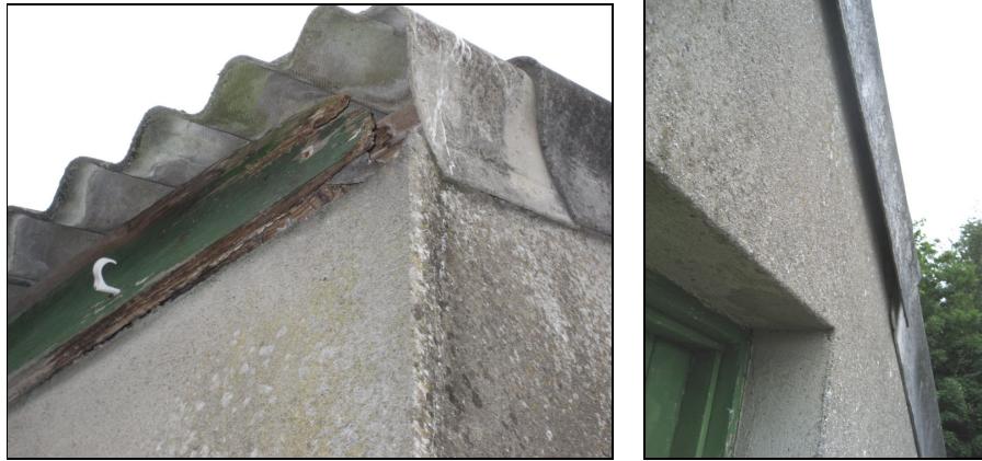
Figure 3: Gaps under lead flashing and under soffit boards can provide access for bats (US Ambassador's Residence outbuildings, Phoenix Park)
