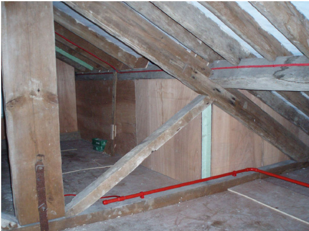
Figure 10: Plywood walls of bat roost zone allowing bats to roost undisturbed (Bishop's Palace, Kilkenny)
